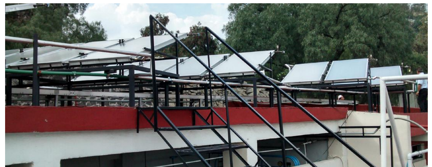
Installation of Solar Water Heating in hospitals in Mexico City.
