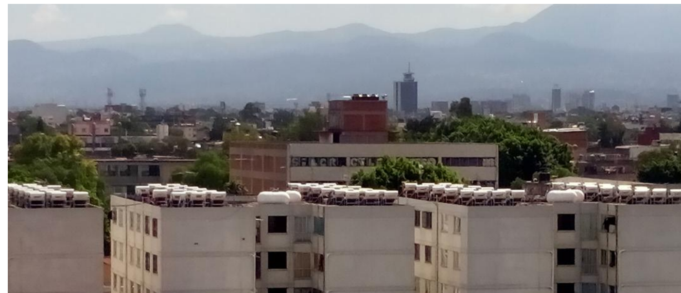
Solar Water Heaters in Mexico City Housing Units.
