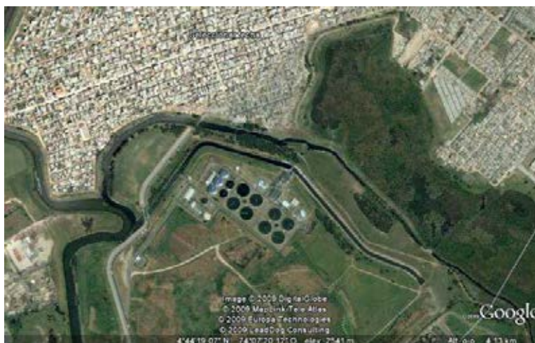
FIGURE 5 THE SALITRE TREATMENT PLANT IN BOGOTA
